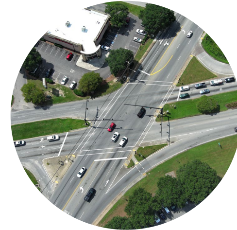
US 52 at Old 52 and Rembert C. Dennis Boulevard
