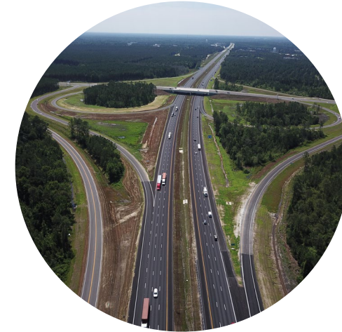
Sheep Island (Nexton) Parkway & I-26 Widening
