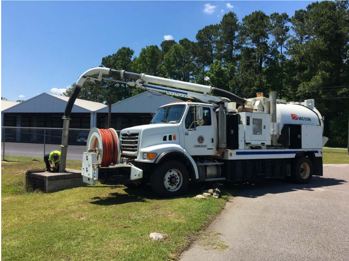
Figure 3-7: Catch Basin Maintenance Operation
