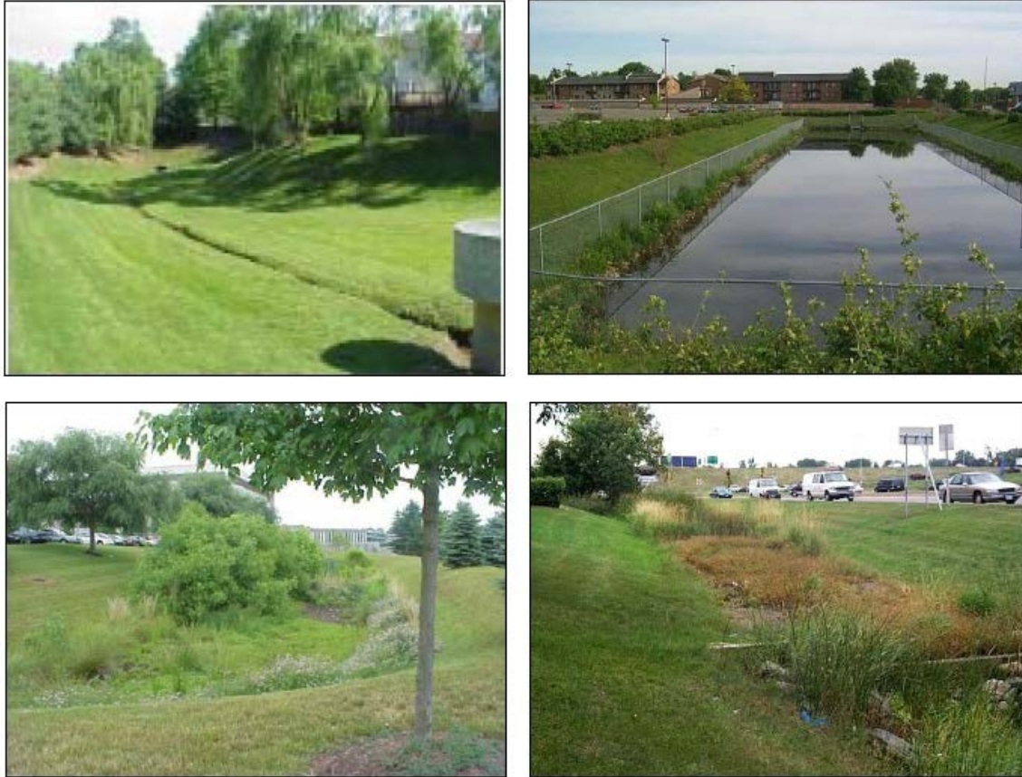
Figure 3-4: Stormwater Best Management Practices (BMPs): (Clockwise from Top Left) Dry Detention Ponds, Wet Detention Ponds, Bioretention Area and Swales
