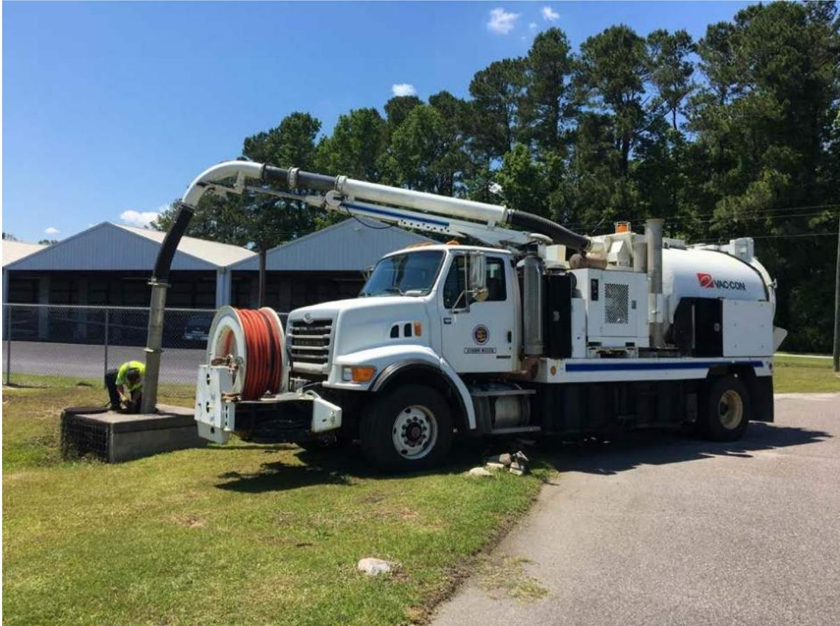
Figure 3-7: Catch Basin Maintenance Operation
