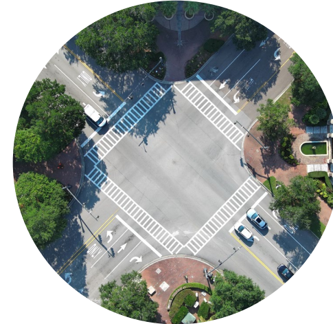
River Landing at Seven Farms Drive
