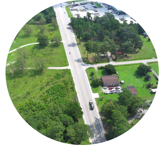
Jedburg Road Phase1
