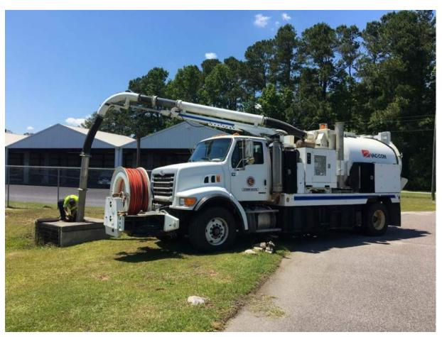
Figure 3-7: Catch Basin Maintenance Operation
