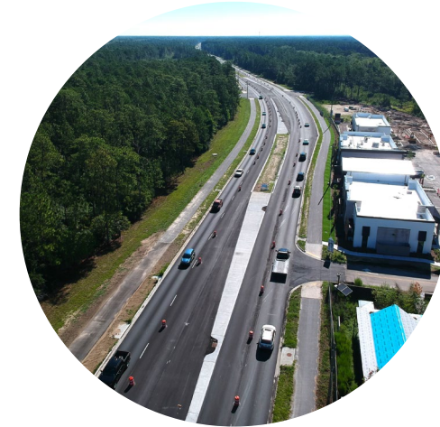
Clements Ferry Road Widening Phase 1
