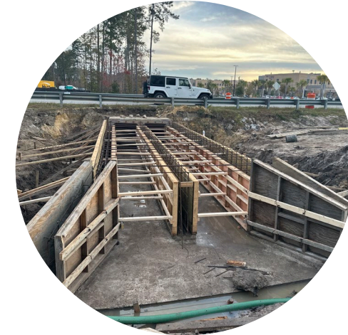
US 176 Widening Phase 1
