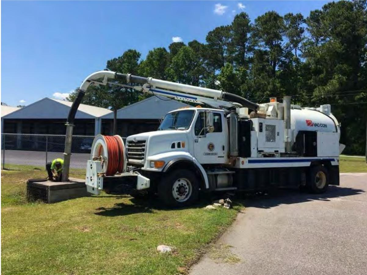
Figure 3-7: Catch Basin Maintenance Operation
